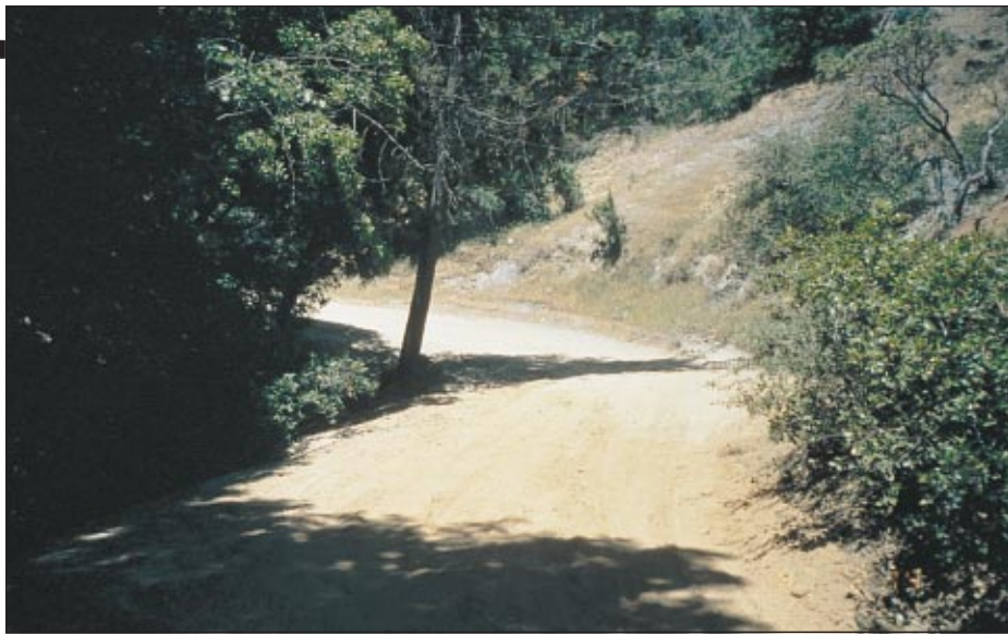
Fig. 1. Old logging roads, such as this one in Whiskeytown National Recreation Area (California), are the primary source of sediment that washes into rivers and streams, degrading habitat for salmon and steelhead trout. To address the problem, the park and Shasta College teamed up to deploy innovative treatments for the restoration of watersheds and habitat recovery. This road was "outsloped" to reduce erosion and sedimentation.
