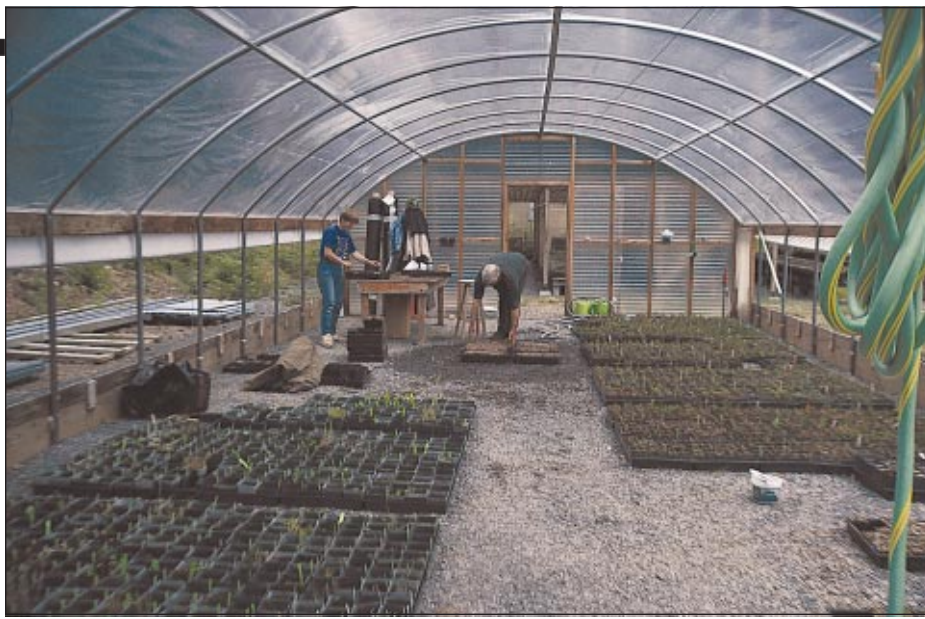
Figure 1. In 1994, Mount Rainier National Park constructed a “coldframe” to serve several purposes. Its primary function is to provide growing space to “harden off” recent transplants (established in the greenhouse) before moving them outdoors to the lathe house. During winter the space is used for stratifying seeds, mixing media, and washing pots. This spring recently potted heathers (2-3 years old) will be moved here.
