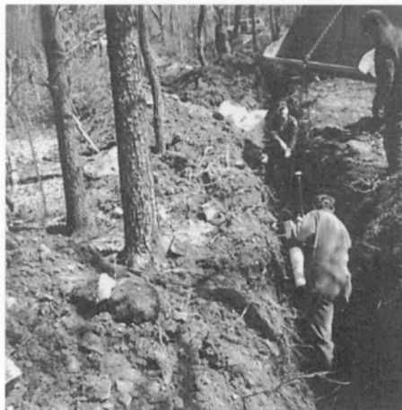
Setting pipe into a ditch. Pipe has no way of slipping.
