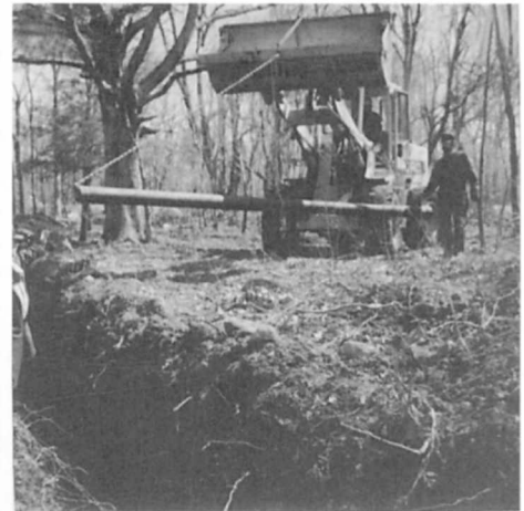
Setting pipe into a ditch. Pipe has no way of slipping.
