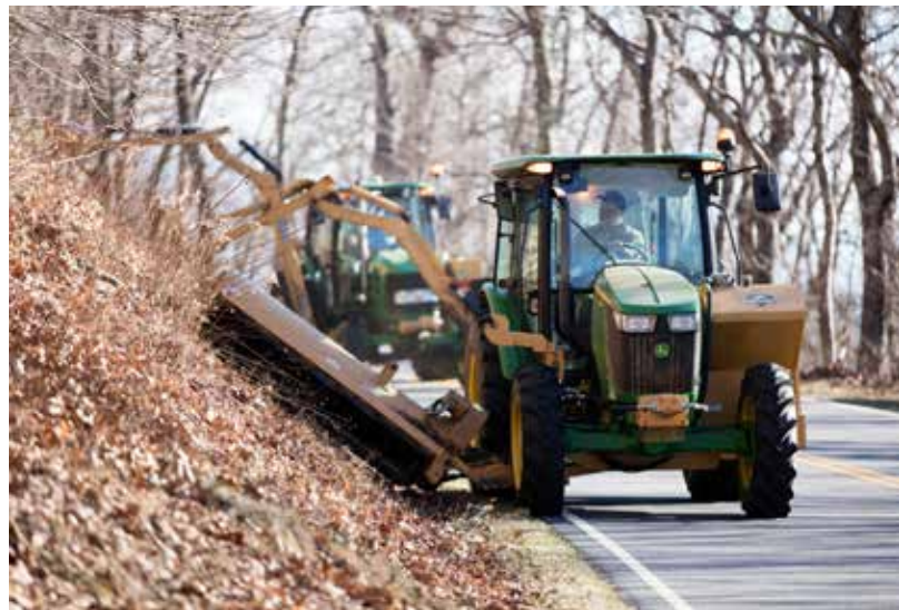
Road crews trim brush along the Skyline Drive in Shenandoah National Park. The Great American Outdoors Act, passed in August, 2020, is helping to fund some $12 billion in deferred-maintenance projects throughout the National Park Service. For Fiscal Year 21, Shenandoah received funding for two projects totaling $29.7 million. NPS Photo
