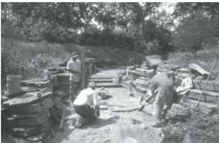
Restoration work underway at the Lily Pool. Courtesy Julia Bachrach.
