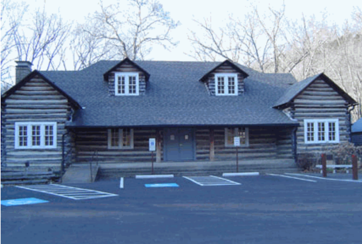
Roadside tavern, existing condition, December 2005.
