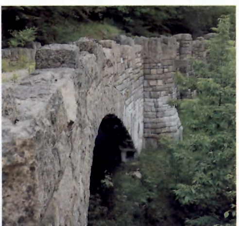
Sixteen stone bridges connect the carriage paths. The first hand-cut granite bridge was built in 1917, the last in 1933.
