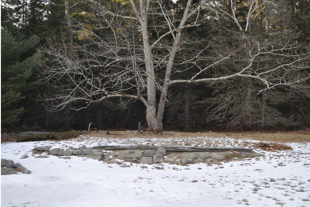
Figure 30. View looking north at the c.1838 barn foundation. (OCLP 2025)
