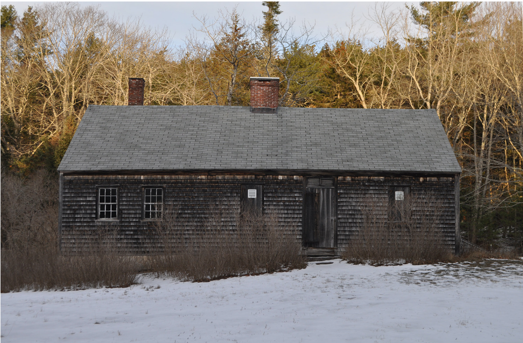
Figure 29. View looking east at the ca.1828/ca.1844 Carroll House. (OCLP 2025)
