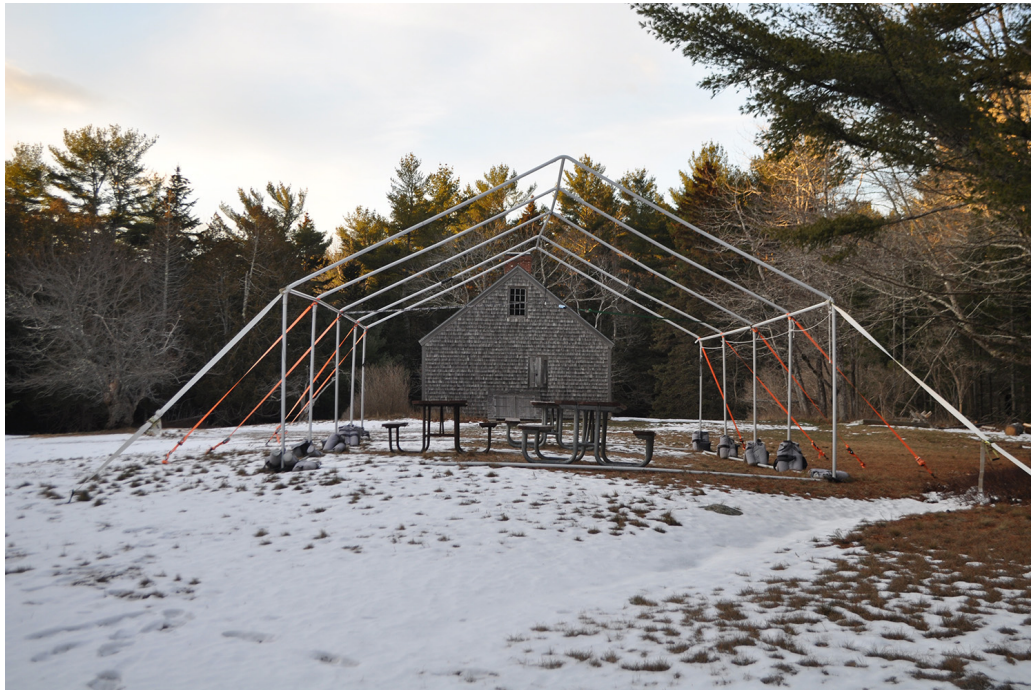
Figure 34. View looking north at the Carroll House and the woods that fill the formerly open fields. In the foreground is the seasonal tent structure. (OCLP 2025)
