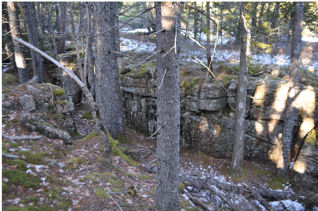
Figure 18. View looking northeast at a portion of “Ma’s Ravine” south of the Carroll House. (OCLP 2025)
