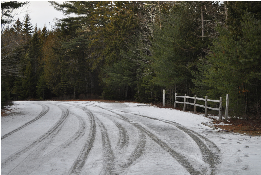
Figure 28. View looking north at the access road and lower parking lot. (OCLP 2025)
