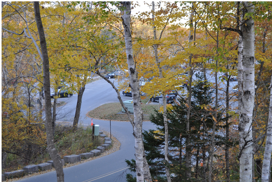
Figure 50. View looking east at the access road and parking lot at Sand Beach. (OCLP 2024)
