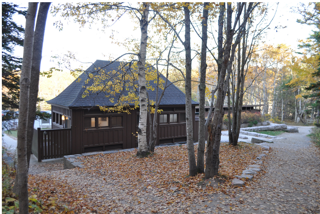
Figure 49. View looking east at the historic Sand Beach Comfort Station, walkways, and retaining walls. The non-historic changing room structure is in the background image right. (OCLP 2024)
