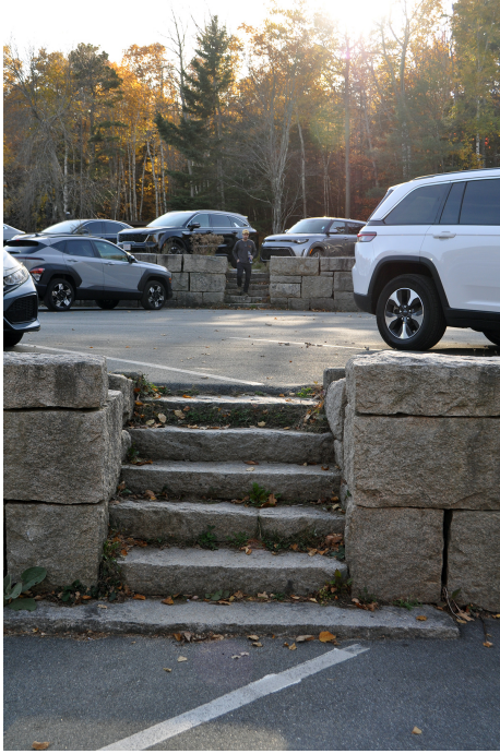
Figure 58. View looking south at steps incorporated into the lower parking lot retaining walls. (OCLP 2024)
