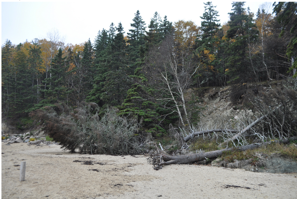
Figure 48. Oblique view at 2024 storm damage along the bluff. View looking northwest. (Acadia NP, 2024)
