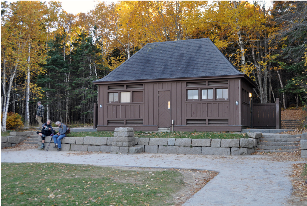
Figure 52. View looking south at the Sand Beach Comfort Station, built in 1952, and stone retaining walls, steps, and drinking fountain that exhibit characteristics of the NPS Rustic Design style. Walkways in this area connect to the lower parking lot, upper parking lot, and the beach. (OCLP 2024)
