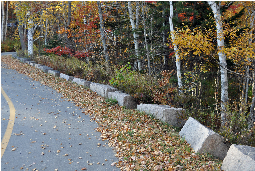
Figure 55. View looking west at rectilinear guardwall stones at the lower parking lot (1955). This NPS Rustic Design style characteristic was introduced on the historic motor road system in the 1930s. Note the woodland vegetation in the adjacent ravine. (OCLP 2024)
