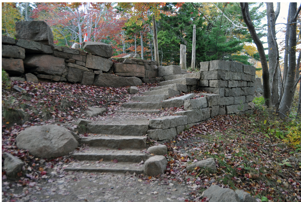
Figure 62. View looking northwest at the stairs at the western end of trail between the upper parking lot and the beach. (OCLP 2024)
