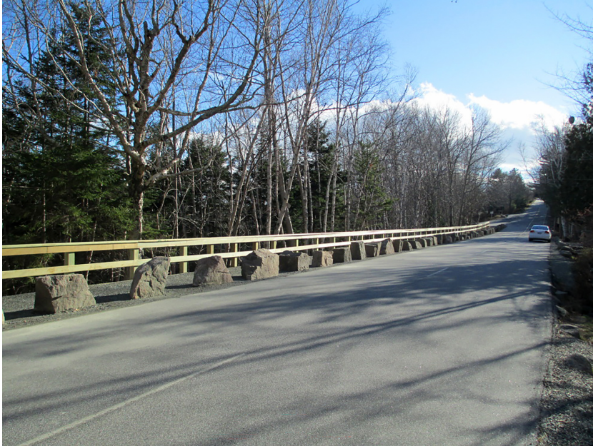
Figure 43. View looking south at the reconstructed Satterlee Trail (trail #9) along Ocean Drive. The Sand Beach Access Road is in the distance at image left. (PEPC, 222534)
