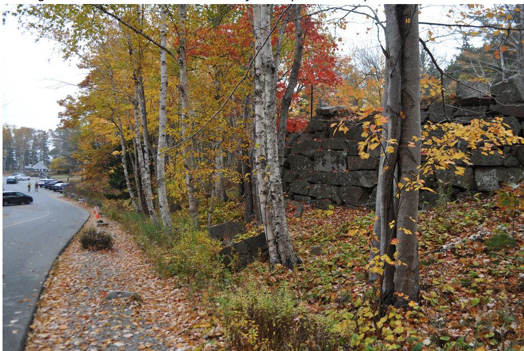
Figure 57. View of the north end of the stone retaining wall that supports the upper parking lot (1934). (OCLP 2024)
