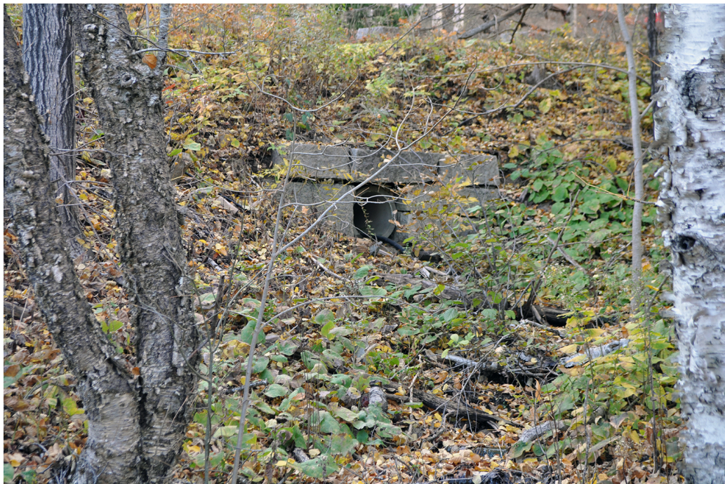
Figure 56. The culvert outlet on the Sand Beach Access Road features a stone headwall, similar to those used on segments of the historic motor road system. (OCLP 2024)
