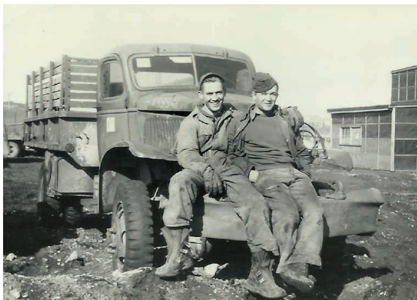
The men of the 807th Aviation Engineering Battalion played a significant role in the building of airfields through the Aleutians.
