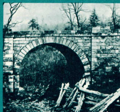
Skew Arch Bridge
