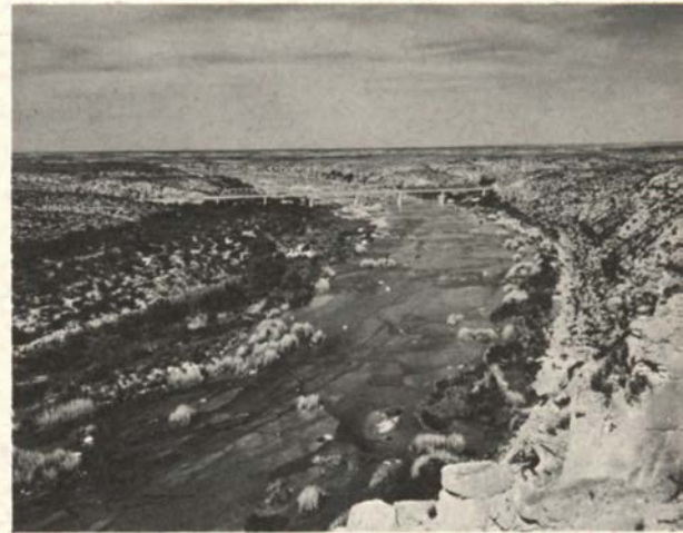
Up Devils River from Diablo East recreation site. Old U.S. 90 bridge will be dismantled. This was one of the finest stream-fishing sites in Texas. When reservoir forms, same resource will be available upstream above Devils Lake.
