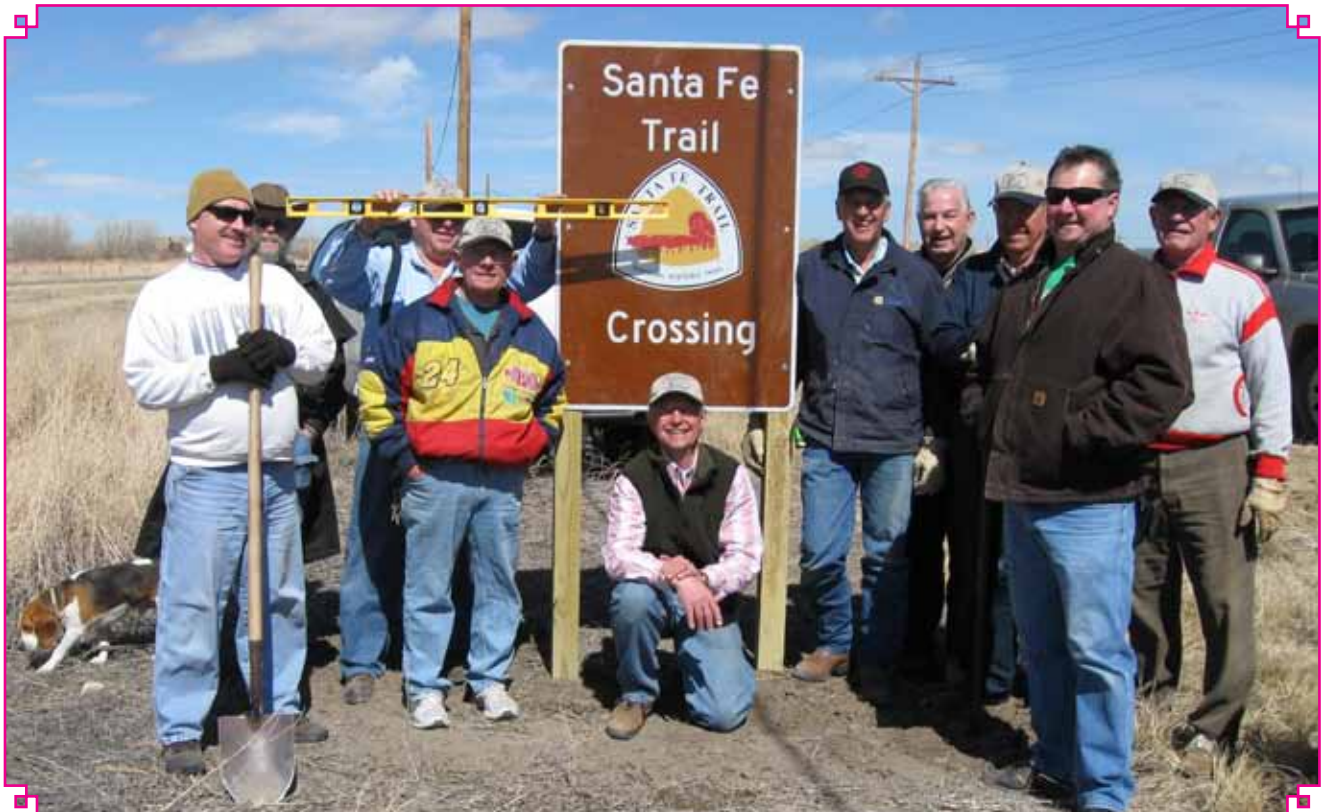
SFTA volunteers help erect a crossing sign in Las Animas County, Colorado
