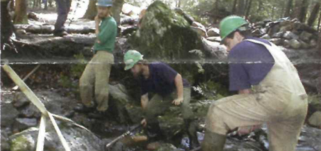
Volunteers repair a section of trail in Maryland. ©NPS
