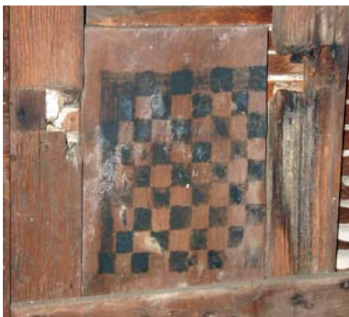
Checkerboard found between wall studs.
