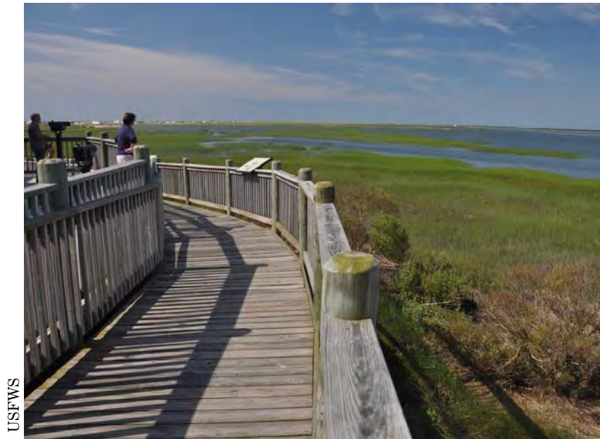
Boardwalk on Refuge
