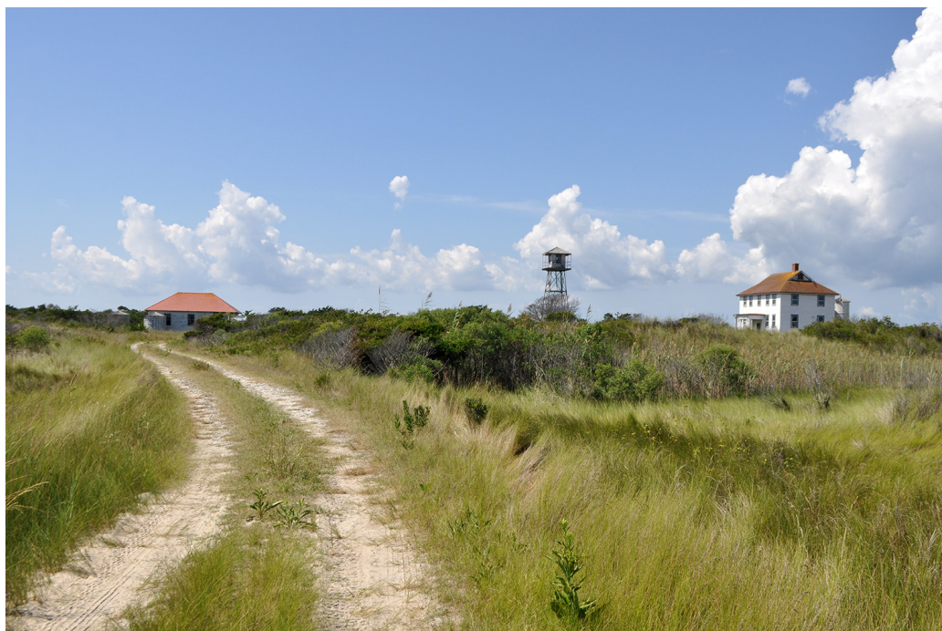
Figure 31. View looking west at the Entrance Road. A grass-covered trace of the Entrance Road segment that once headed northwest is visible at image right. (OCLP 2023)
