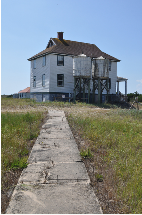
Figure 35. View looking southwest at the concrete walk that connects the Generator House to the Station House. The two water cisterns collected water from the Station House roof. (OCLP 2023)
