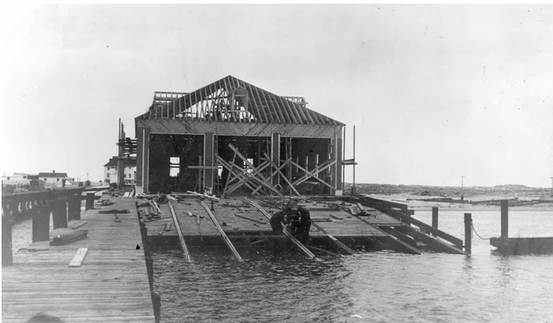
Figure 15. Boathouse construction in 1938 at the wharf. (USCG Archives, Washington DC, from CLI 2004: 44)
