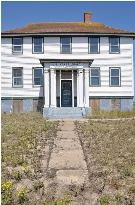
Figure 34. View looking north at some of the concrete walkways at the Station House. (OCLP 2023)
