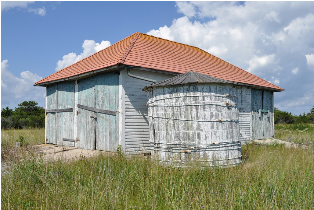
Figure 39. View looking northwest at the Garage/Boathouse and cistern, built in 1922. (OCLP 2023)
