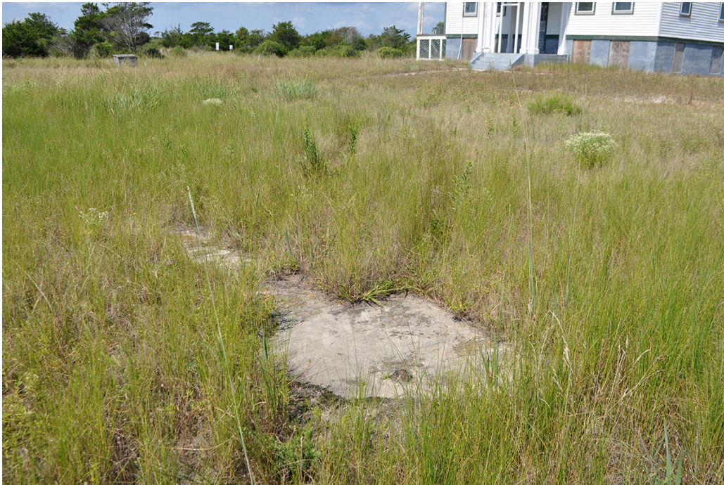
Figure 41. View looking northwest at the foundation of the flagpole that appeared in a 1962 photograph. (OCLP 2023)
