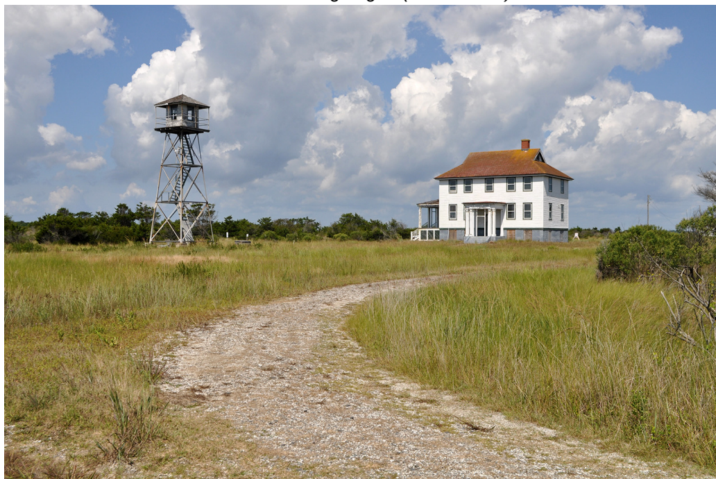
Figure 32. View looking northwest at one of the roads in the station grounds. (OCLP 2023)
