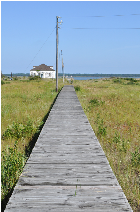
Figure 28. View looking north at the 1930s facilities built north of the Station House. (OCLP 2023)
