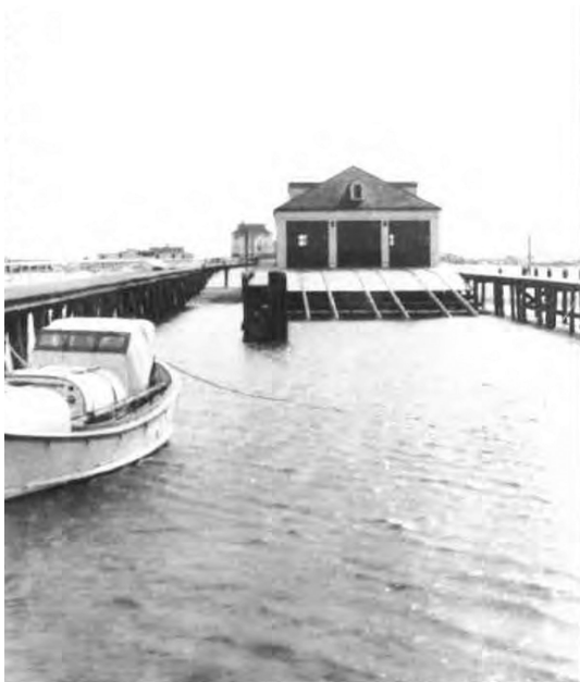
Figure 17. View looking south at the wharf and the completed boathouse, c.1939. In the background is the station house (to immediate left of boathouse) and other unknown buildings. (USCG Archives, Washington DC, from CLI 2004: 45)
