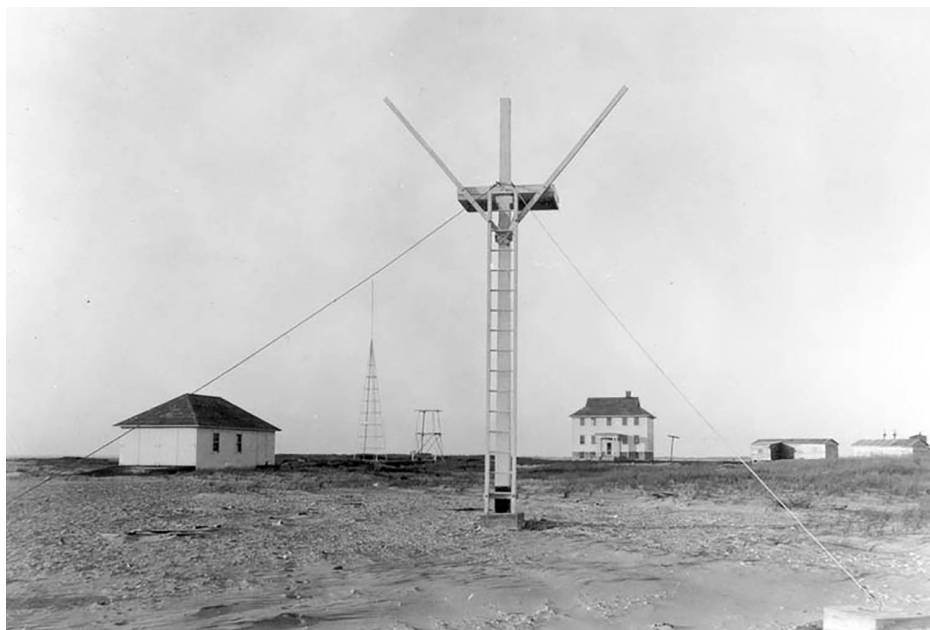
Figure 12. A c.1922-1923 photograph of the station complex looking north. From image left to right are the boathouse/garage, station house, and factory buildings. The structure in the foreground is a wreck pole. One of the two towers in the background is shown on the 1925 map, but it is unclear which one: the taller tower is a signal/flag tower while the shorter tower is the two-story lookout, prior to addition of a cabin. (USCG archives, Washington DC, from CLI 2004: 43)
