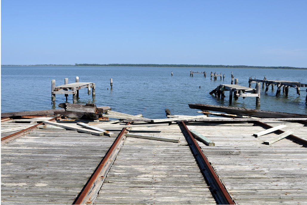
Figure 38. View looking north-at the marine rail launchway and flanking finger piers, built in 1931-1935. In the background at image right are the remnants of the wharf and T-dock. (OCLP 2023)
