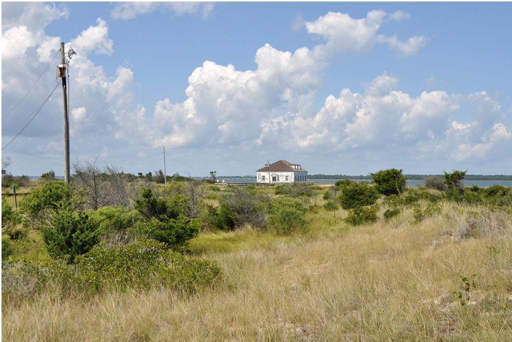
Figure 29. View looking north-northwest toward the Boathouse at Toms Cove. Traces of now-vegetated dunes (image right) are still visible along the sand fence northeast of the Station House. (OCLP 2023)
