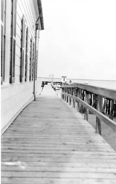
Figure 18. View looking north at the boathouse, and walkway, c.1938. At image right is the wharf and bulkhead, and the pumphouse at the end of the wharf. (USCG Archives, Washington DC, from CLI 2004: 45)
