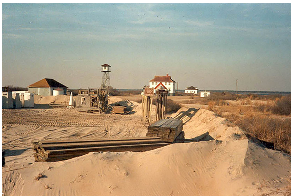
Figure 25. View looking north from "maintenance yard" created by park staff in the 1980s. (Courtesy of Mel Olsen, Assateague Island NS)
