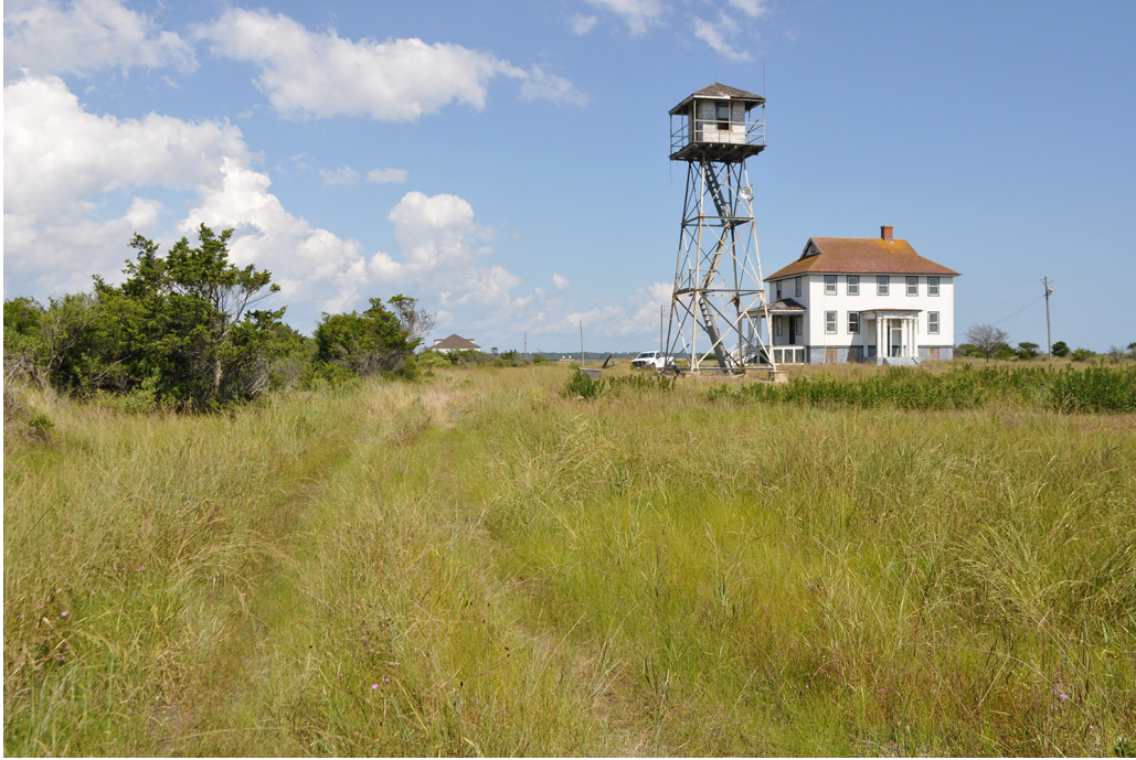
Figure 33. View looking north at one of the roads in the station grounds. (OCLP 2023)
