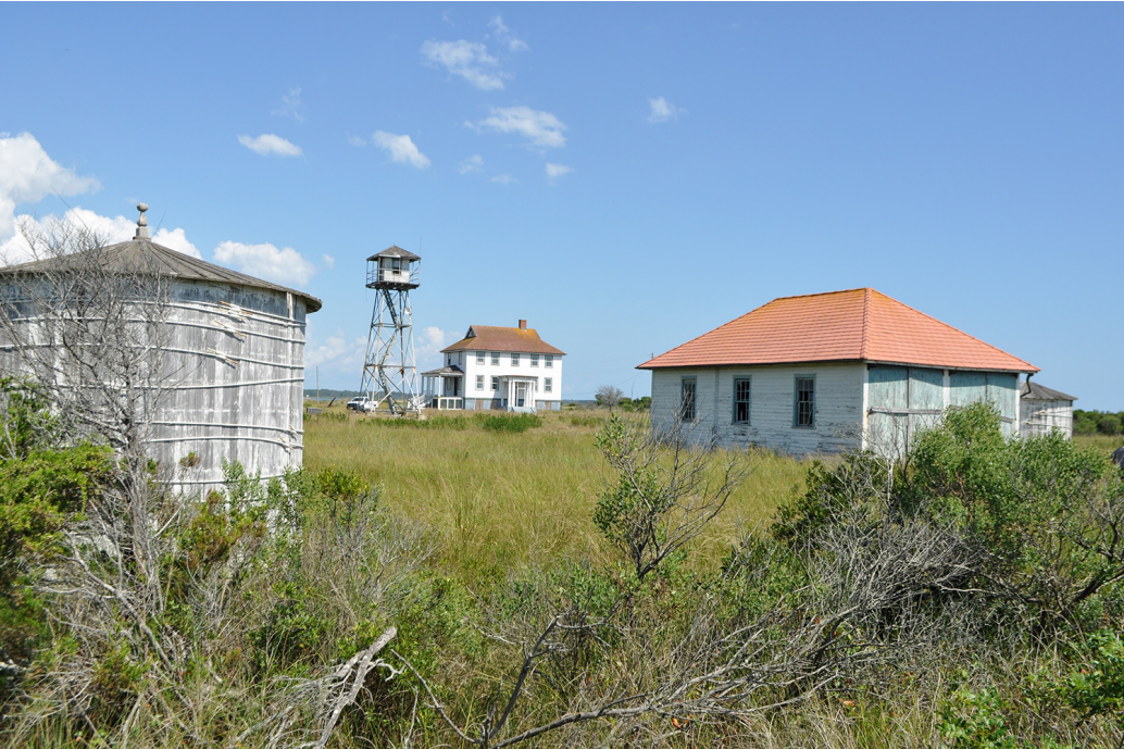
Figure 30. View looking northeast showing a transition from shrubland to grasses. The water cistern at image left was formerly located on the west side of the new boathouse. (OCLP 2023)
