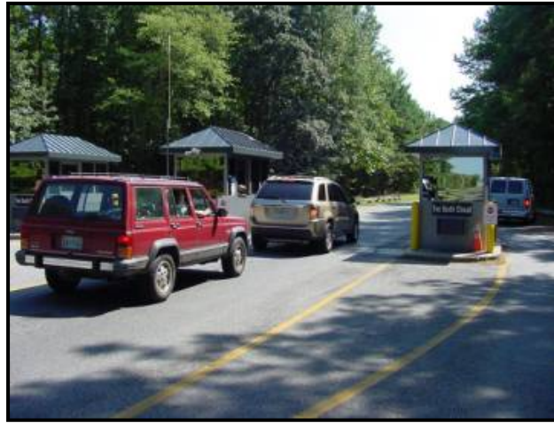
Figure 3-33. Chincoteague NWR Entrance Booths (USFWS refuge Web site)
