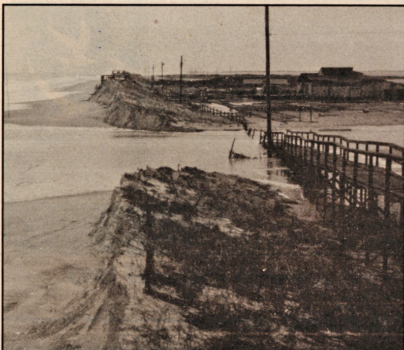
Dune damage showing the narrow winter beach from the January 4th storm near parking lot 3 in Virginia.
