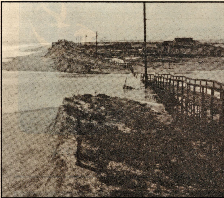
Dune damage showing the narrow winter beach from the January 4th storm near parking lot 3 in Virginia.
