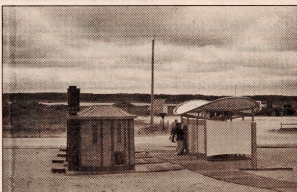
Portable, solar powered visitor comfort station in Virginia District
