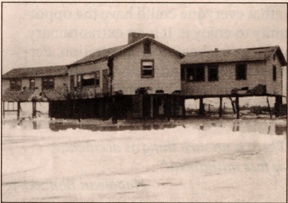
- McCabe beach house after 1992 storm.
