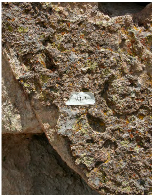
Figure 5. Edge of an erosional remnant of a Type 7 case hardened surface showing a more recently exposed adjacent surface (left) that is less altered.
