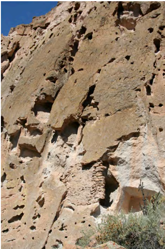
Figure 3. Cavate B002 with its surviving masonry wall (bottom center). Note the broad range of case hardened surfaces of the surrounding tuff, and the "swiss-cheese" texture that develops where the durable case hardened surface is breached, exposing the soft underlying tuffs to erosion. The extensively altered surfaces (upper half) are Types 6 and 7 (see Table 1); on the far right a more recently exposed surface, slightly recessed and having a smoother texture, has developed another rind. Areas of recent erosion appear as white or grey patches (Type 1); erosion at the lower right edge of the cavate threatens to undermine the prehistoric wall. Some of the freshly exposed tuff has begun to acquire silt-clay coatings (Type 2) that constitute one of the initial stages of case hardening. At bottom left, moderately well indurated surfaces have silt-clay layers colonized by lichens and other microflora (which appear yellow, green and black in the photo). Note the partially detached boulder above the wall, the column of cantilevered stones at the east end of the surviving wall, and the erosion of the tuff just below this column.
