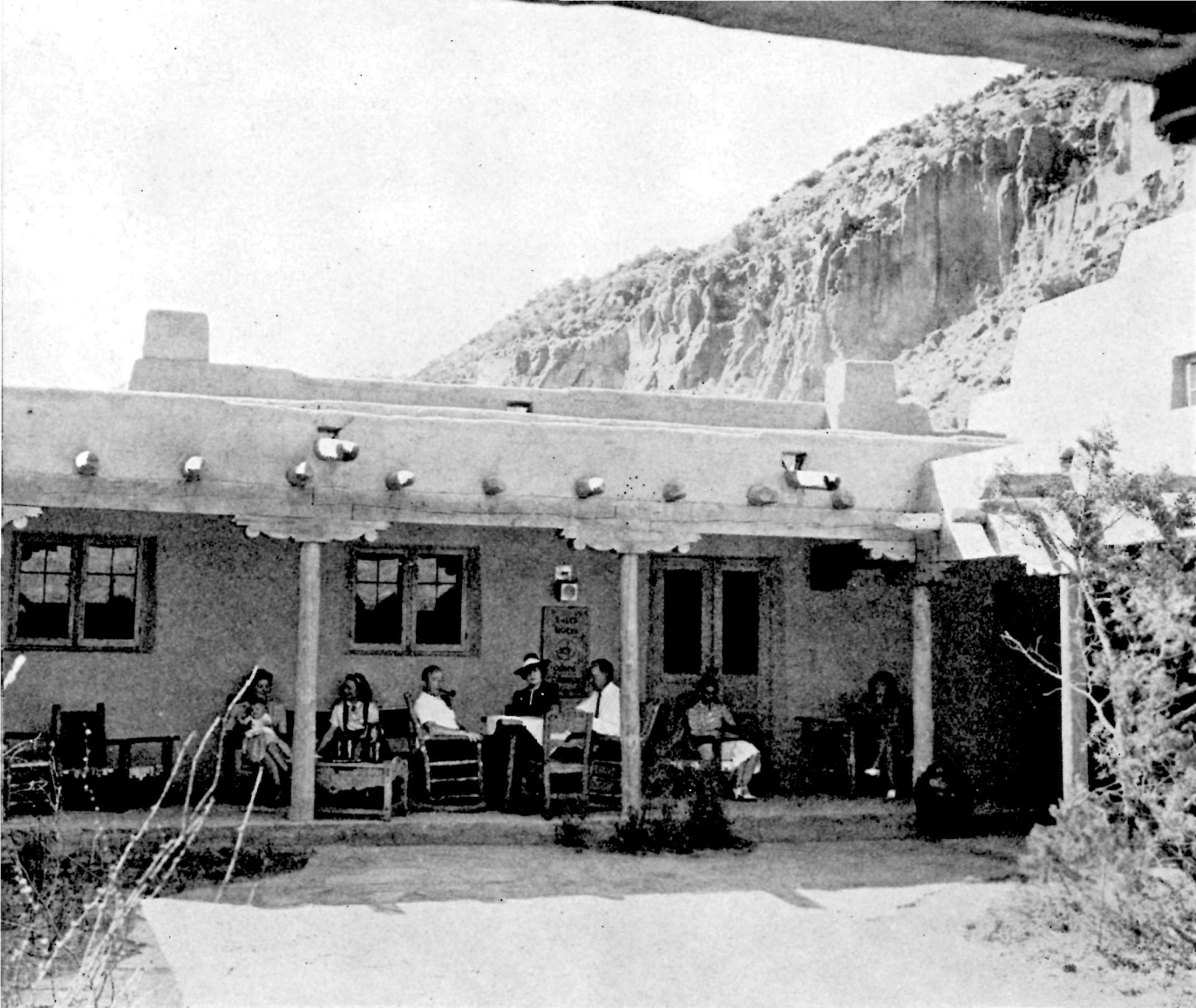
The new lodge in the heart of the canyon
