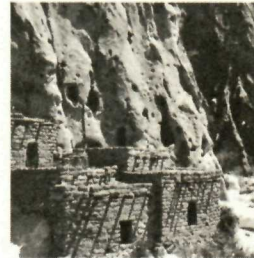
RESTORED TALUS HOUSE
