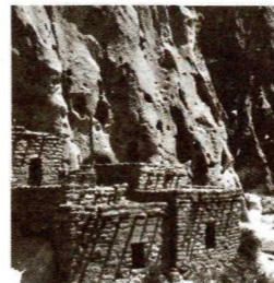
RESTORED TALUS HOUSE
