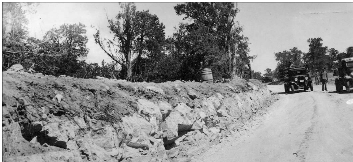
Construction of the entrance road into Frijoles Canyon, 1933
