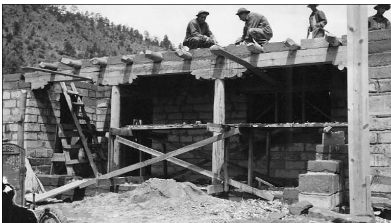
Construction of Frijoles Canyon Lodge
