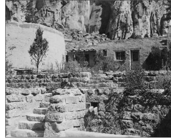
CCC Lodge and "Kiva"
