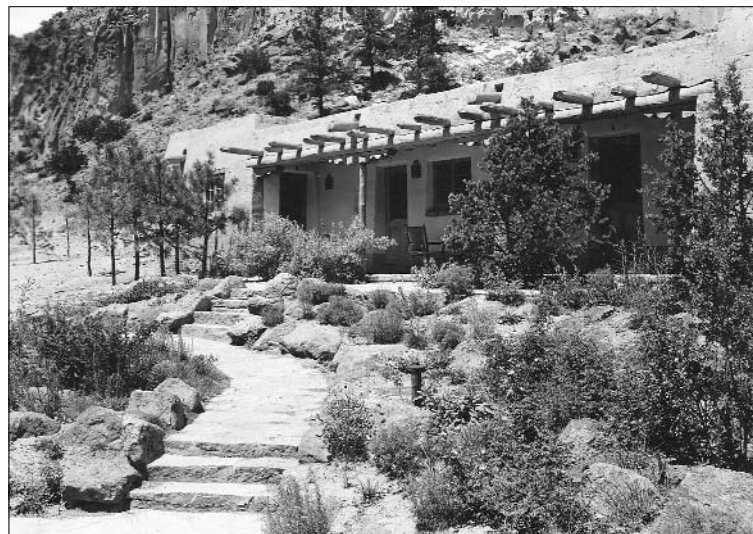
CCC cabins Frijoles Canyon Lodge 1940. Now used as staff quarters.
