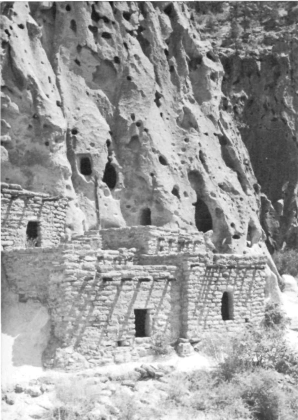
Restored Talus House.
