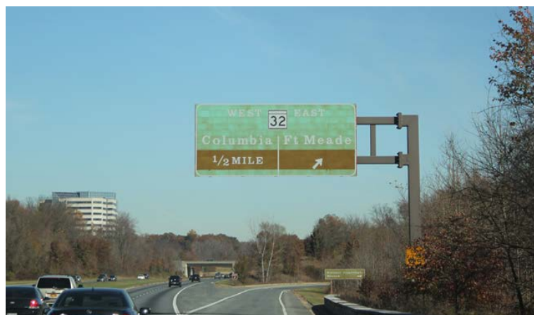
Figure 1: An exit sign not in compliance with the MUTCD.
