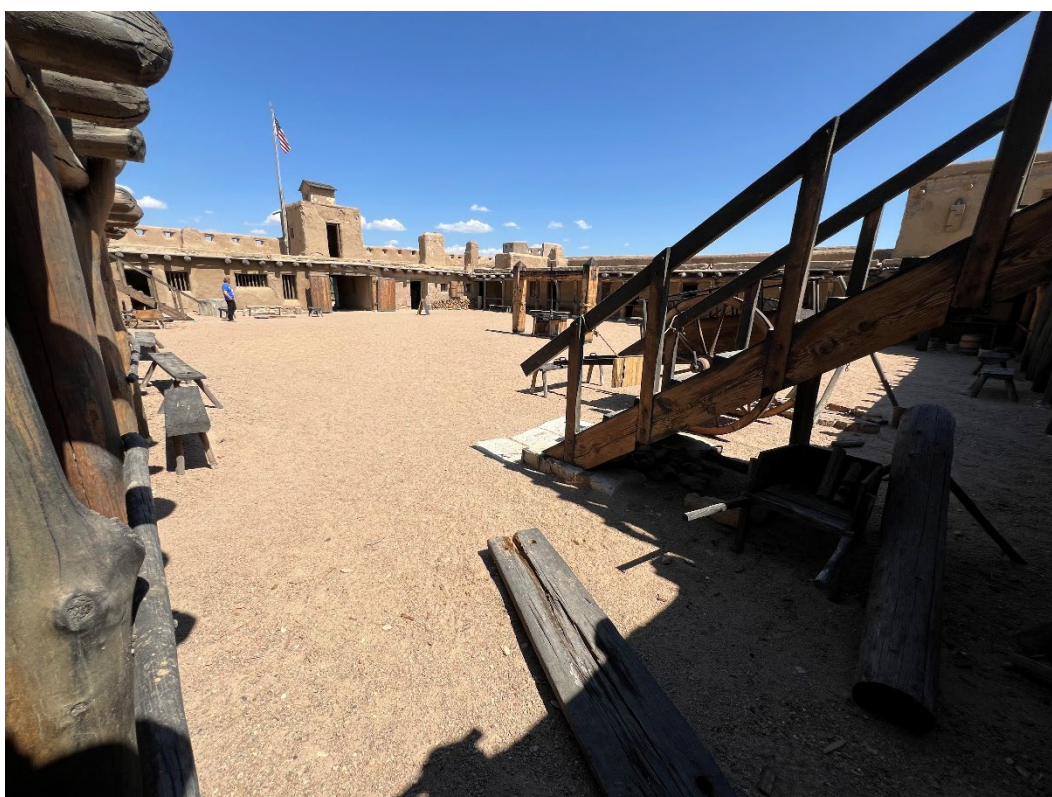
Photo Number: 50T.1728_14 Description: View of the interior plaza from the lower level. View: East
