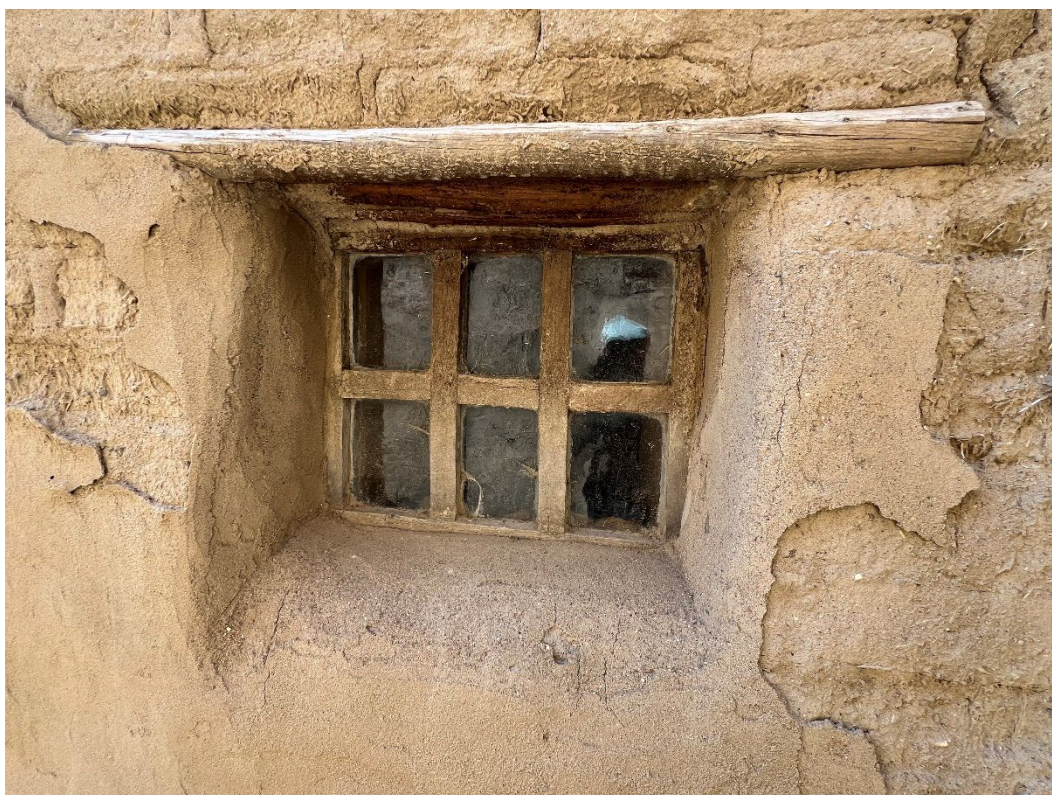
Photo Number: 50T.1728_24 Description: Another example of window showing a six-lite window. View: Detail
