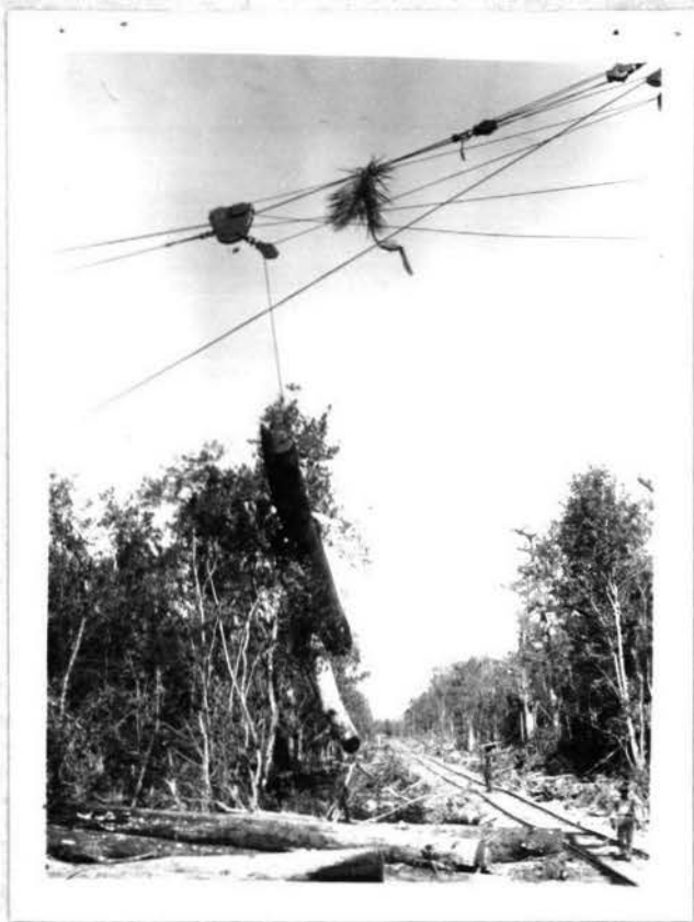
Overhead skidder bringing log out of the woods.
