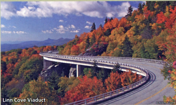
Linn Cove Viaduct
