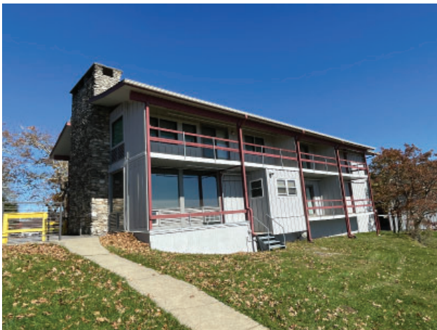
HW0647_Mount Pisgah Inn Lodge and Office_10-24_ars_09
