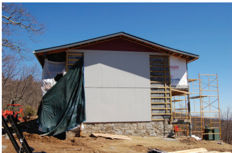
Figure 42. (Top) Unit C in the early days of the 2008 renovations. (Blue Ridge Parkway)
