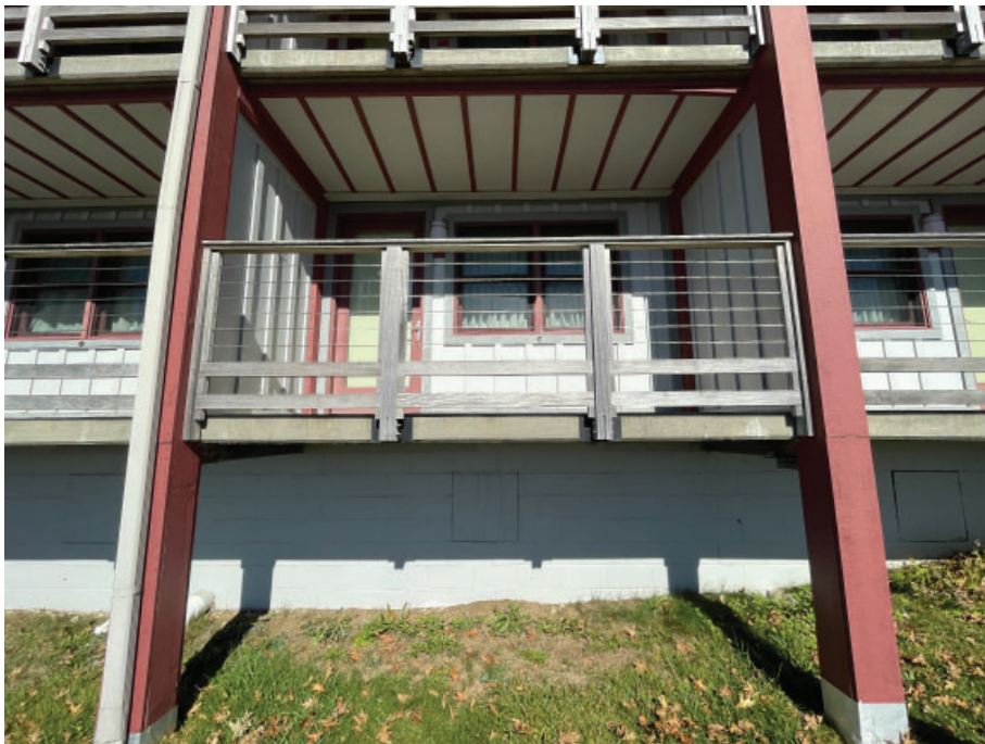
Figure 62. The replaced railings at Unit C are weather-resistant unpainted wood (Brazilian walnut) and stainless steel cable, as shown in this image of a typical bay on the balcony side of the building. (NPS)
