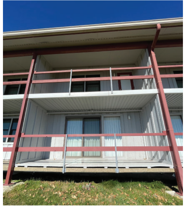
Figure 55. (Left) Typical bay at north side of Unit B. (NPS)
