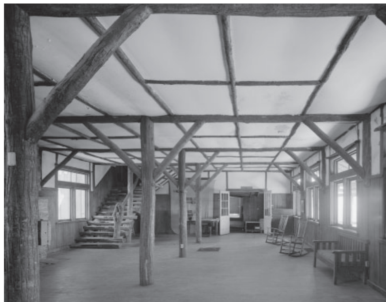
Figure 38. The lobby of Pisgah National Forest Inn's main lodge, 1987. (Photographed by J. Weiland for NPS, HABS NC-356-28. https://www.loc.gov/pictures/item/nc0431.photos.212312p/ )
