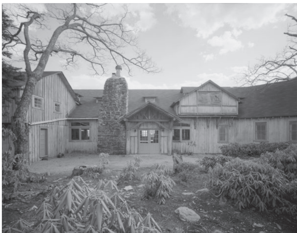
Figure 12. Pisgah National Forest Inn's main lodge, photographed in 1987 by J. Weiland for the Historic American Buildings Survey. (Library of Congress, HABS NC-356-12. https://www.loc.gov/pictures/item/nc0431.photos.212296p/ )
