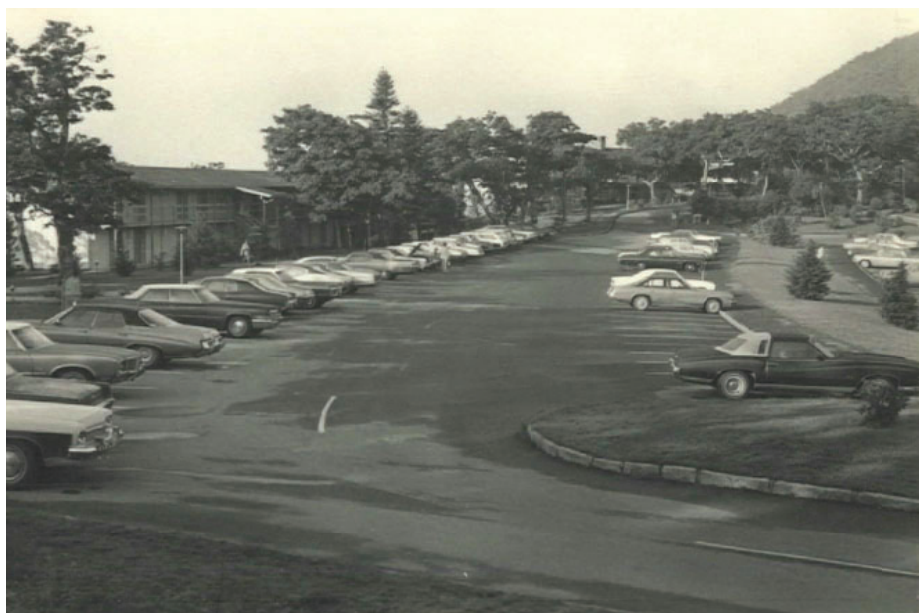
Figure 36. The parking lot and buildings at Pisgah Inn, August 1973. Photographed by C. E. Westveer. (NPS, Blue Ridge Parkway Archives)
