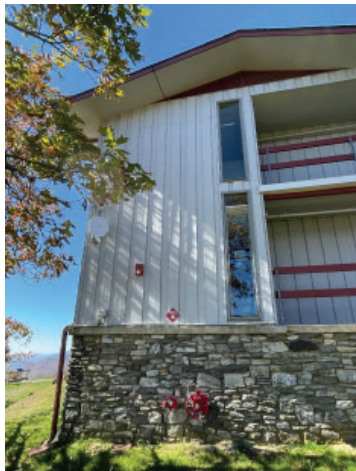
HW0647_Mount Pisgah Inn Lodge and Office_10-24_ars_05
