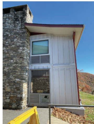
HW0647_Mount Pisgah Inn Lodge and Office_10-24_ars_10
