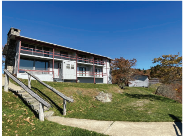
HW0647_Mount Pisgah Inn Lodge and Office_10-24_ars_08
