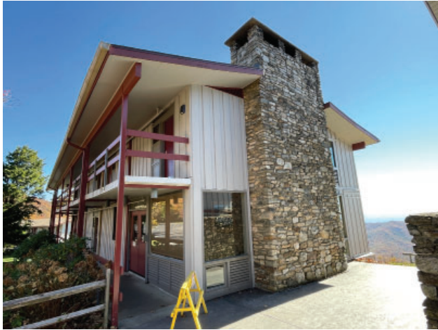
HW0647_Mount Pisgah Inn Lodge and Office_10-24_ars_01
