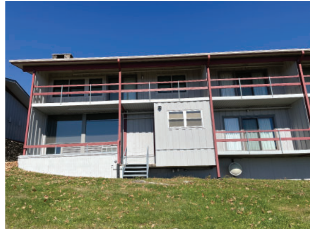
Figure 49. (Right) Rear view of the Lodge showing the rear addition and changes to the fenestration patterns from original construction. (NPS)
