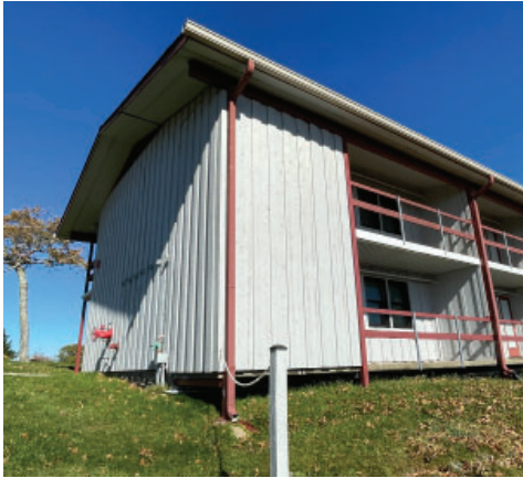
Figure 52. Building enclosure at utility rooms at south corner of motel Unit B. (NPS)
