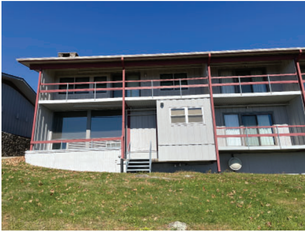
HW0647_Mount Pisgah Inn Lodge and Office_10-24_ars_07
