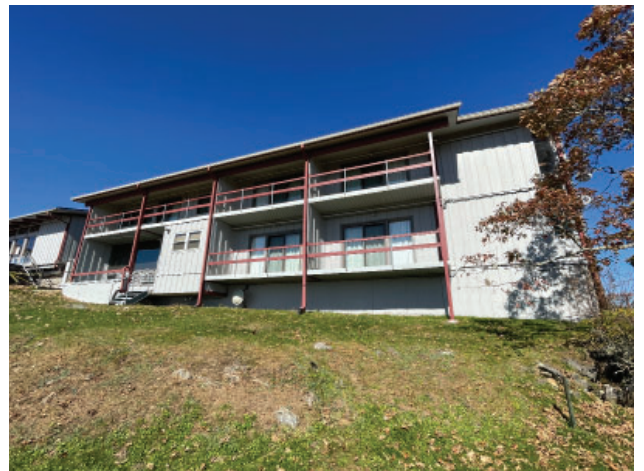
HW0647_Mount Pisgah Inn Lodge and Office_10-24_ars_06
