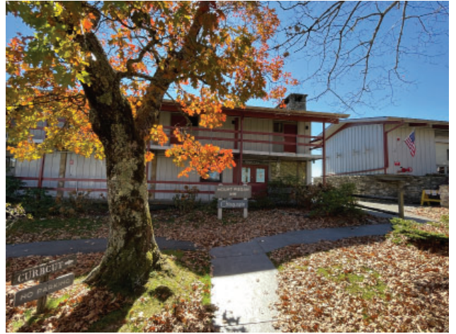
HW0647_Mount Pisgah Inn Lodge and Office_10-24_ars_02
