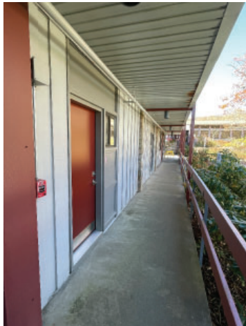
HW0647_Mount Pisgah Inn Lodge and Office_10-24_ars_03
