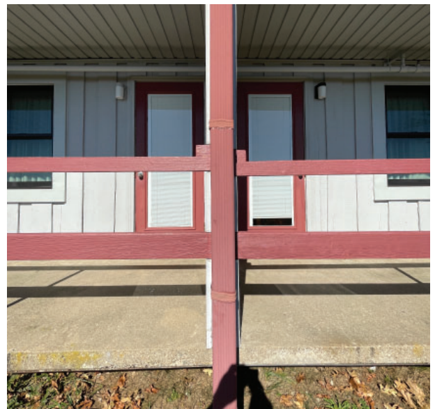
Figure 57. Modifications to top rails at the balcony side of Unit B. (NPS)
