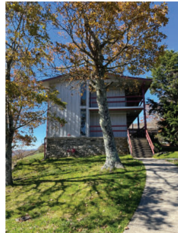
HW0647_Mount Pisgah Inn Lodge and Office_10-24_ars_04
