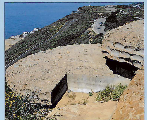
Fire control stations helped batteries direct their gunfire. The top bunker served as a battery command post. The bottom bunker was used as a base-end station,
