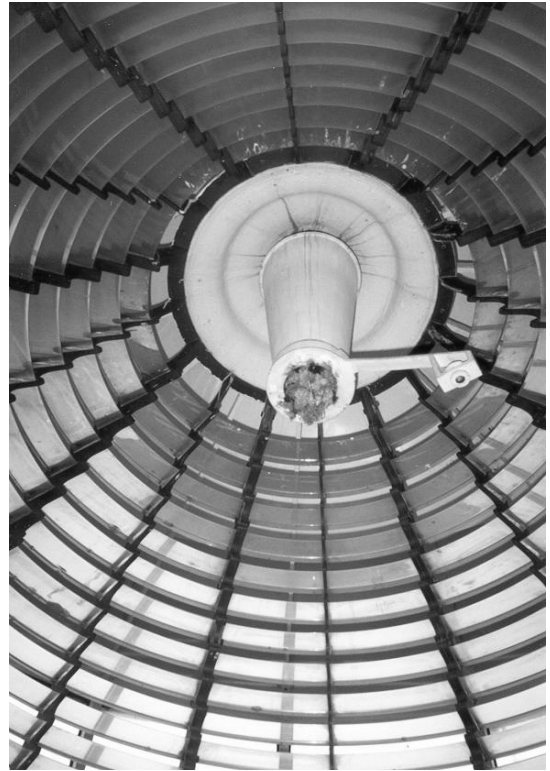
Figure 45 Detail of Fresnel lens.
