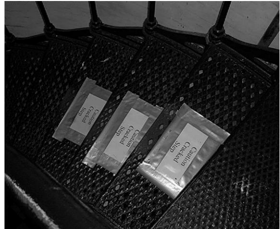
Figure 29 Three treads with notable cracks, below Landing #1.
