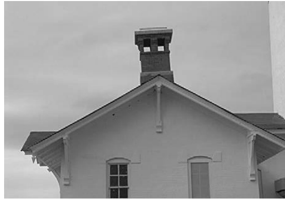
Figure 28 South chimney above the Oil Room.
