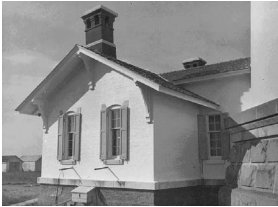
Figure 19 Photo of south elevation by U.S. Coast Guard, 1948.
