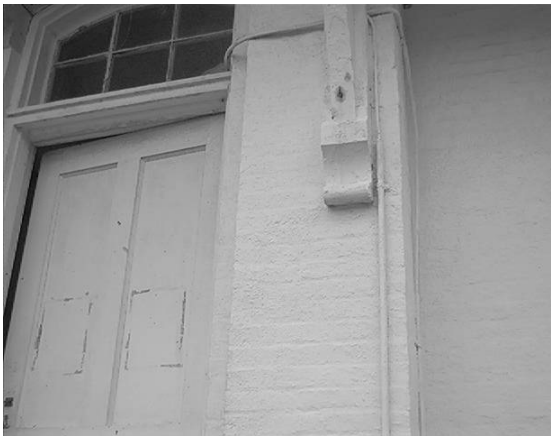
Figure 37 Detail of utility routing through door frame
