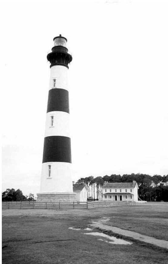
Figure 3 Bodie Island Light Station, looking south, 2002.
