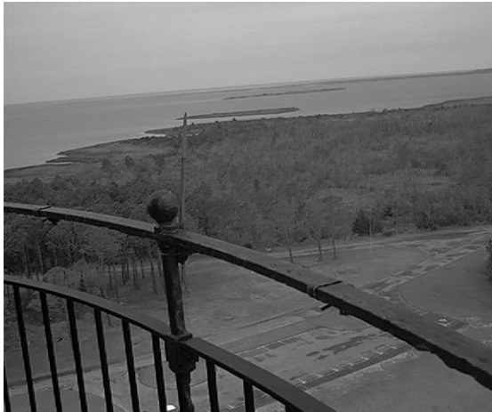
Figure 41 Lightning rod installed on gallery handrail.
