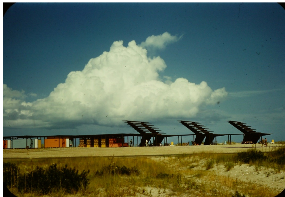
Sun shades and the colorful bathhouse at the Coquina Beach Day Use Area.
