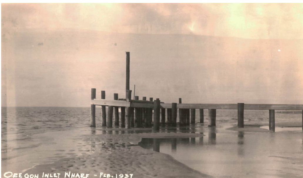
OREGON INLET WHARF - FEB. 1937
