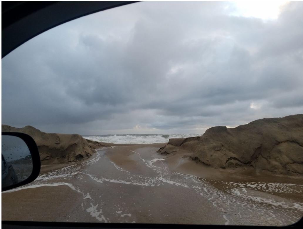
Dune breach north of Rodanthe, NC around high tide this morning.
