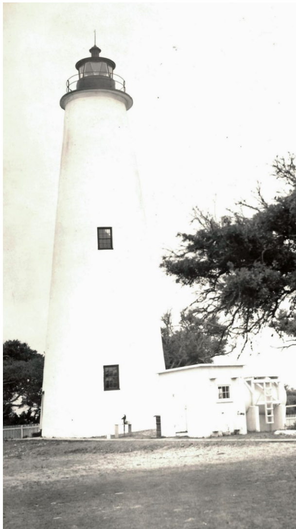
Ocracoke Lighthouse on May 29, 1941. Notice the black trim on the window sashes and the exterior parge finish of the lighthouse before the application of the thick shotcrete coating (sometimes called gunite) in the early 1950s.
