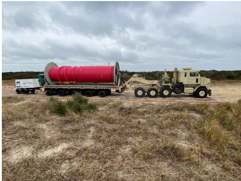
Large cable reel for the Pole Road underground power line project.
