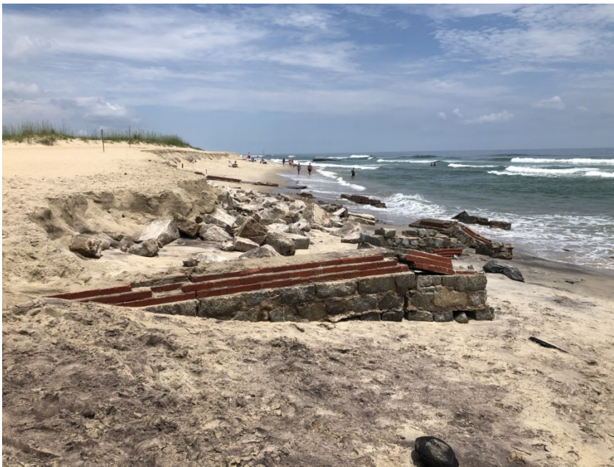
Photo of the fence foundation on July 1, 2020.
