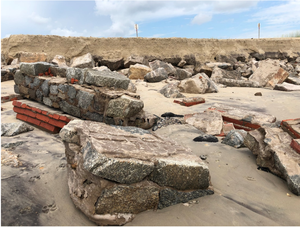
Photo of the fence foundation on July 1, 2020.
