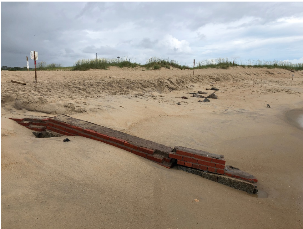
Photo of the fence foundation on July 8, 2020.
