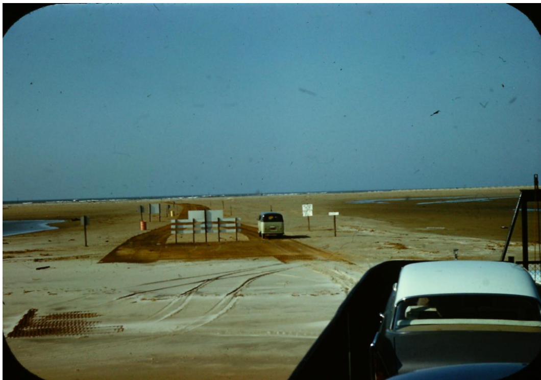
Cape Hatteras National Seashore's bus can be seen traveling on pierced steel planking at the north end of Ocracoke Island in this 1960s photo. The planks, also know as Marston mats, were used during War War II to provide reliable transportation over all kinds of terrain. The nickname came from Marston, N.C., where the planks were first used in 1941. In the foreground of the photo, a vehicle is waiting on a ferry.
