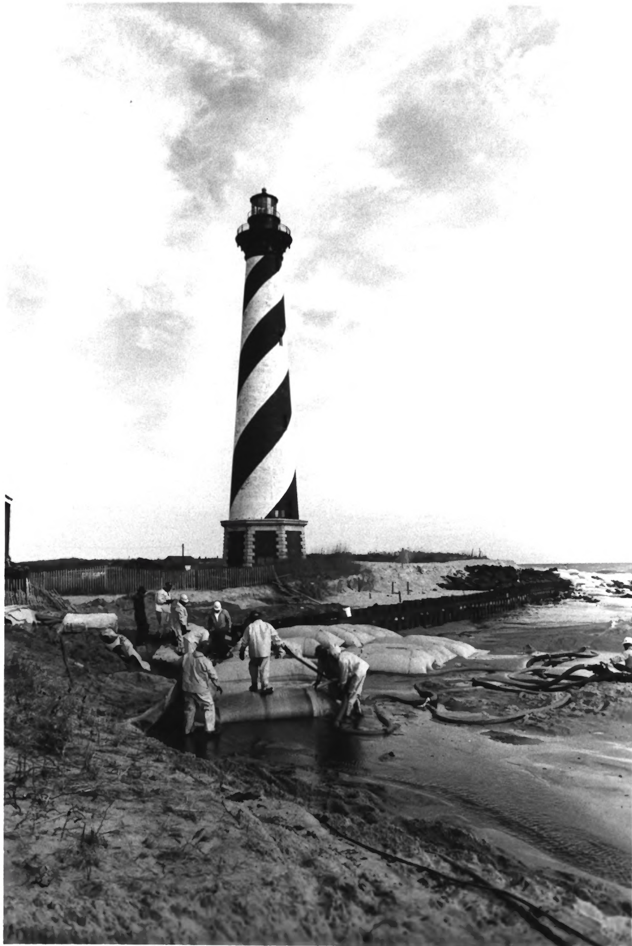
Cape Hatteras Light Station Buxton, NC Park staff fill sandbags after 1994 storm NPS photo by Candace Clifford, 1994
