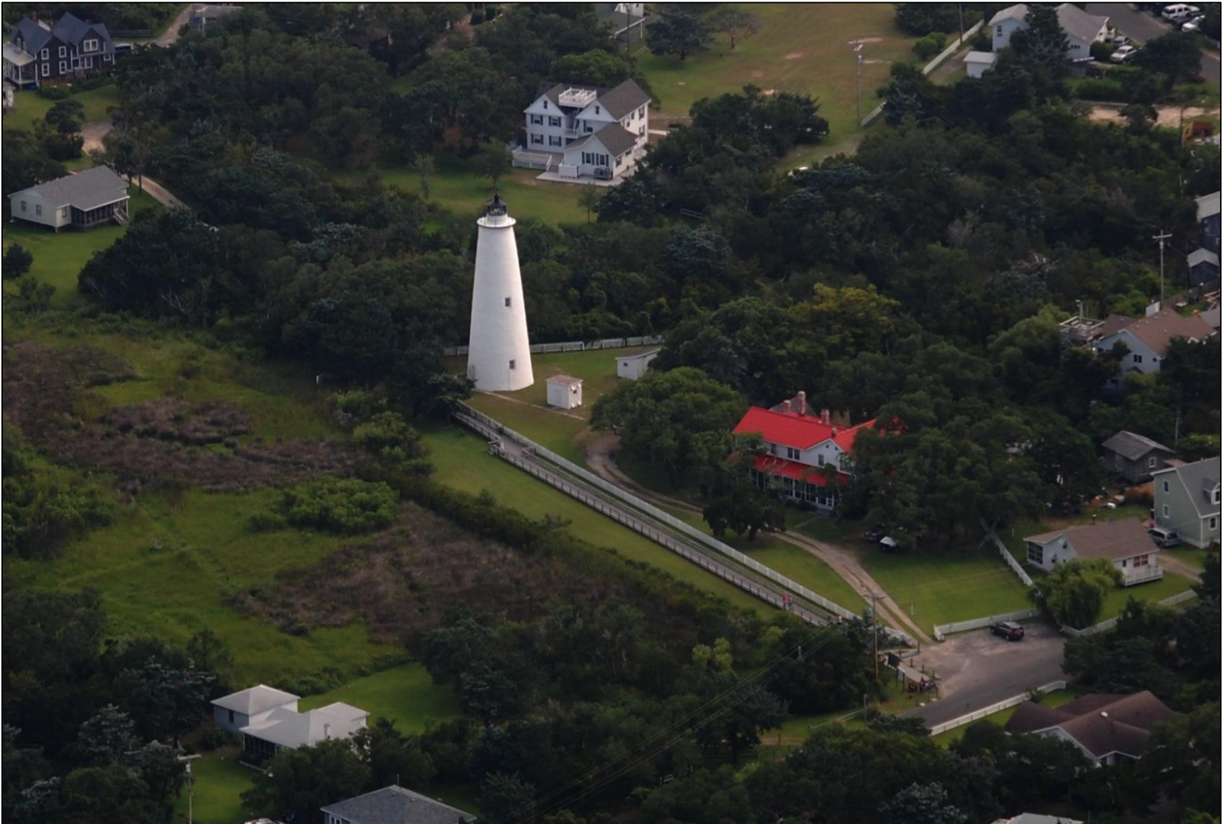
Figure 2. Aerial Image of the Ocracoke Light Station, 2105
