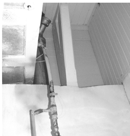
Figure 73 View of large bracket behind and above shower, installed to support water tank at second floor. Note original cornice on rear wall. (NPS-SERO-CRS, 2002)
