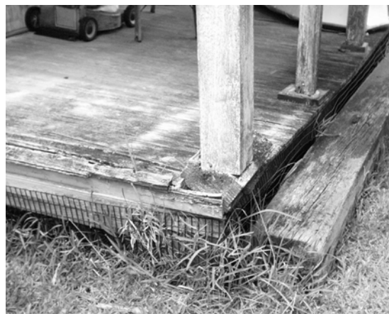
Figure 60 View of northeast corner of front porch, showing corner post seriously destabilized by deterioration of the sills at that location. (NPS-SERO-CRS, 2002)
