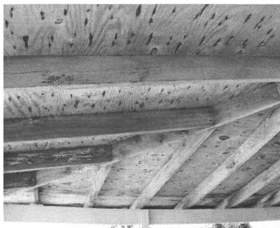
Figure 22 View of original porch roof framing at north corner of house. (NPS-SERO-CR, 2003)
