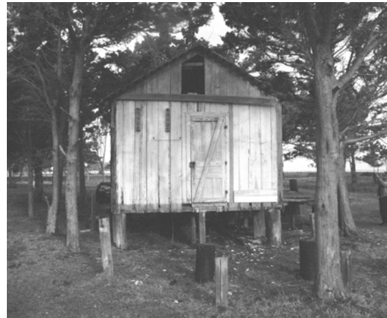
Figure 5 View of southwest end of house; note piers in foreground which supported the modern addition that was removed after 1984. (NPS-SERO-CRS, 2001)
