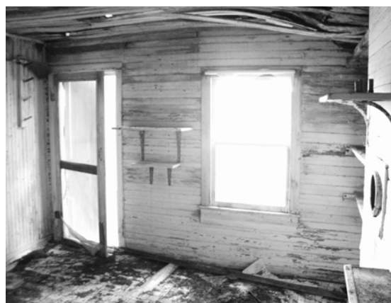
Figure 13 View west in main room. (NPS-SERO-CRS, 2001)
