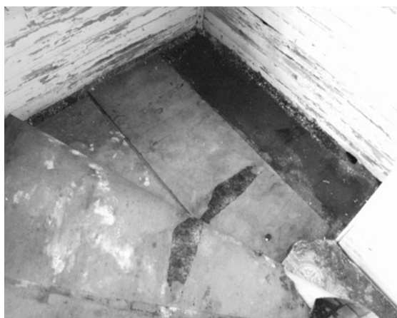
Figure 15 View of floor in northwest corner of main room, showing early felt-based, imitation linoleum under two later floor coverings. (NPS-SERO-CRS, 2001)
