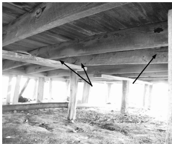
Figure 7 View of floor framing; arrow at right indicates where joist has split; arrows at center show location of two joists that have broken where they cross the added support beam. (NPS-SERO-CRS, 2001)
