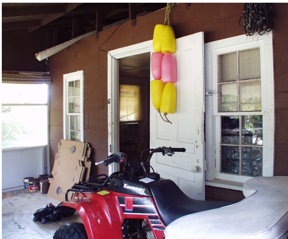
Figure 25 View of front porch with original windows and door. (NPS- SERO- CRS, 2002)
