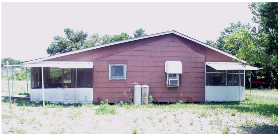
Figure 23 View of southwest side of house, showing line of original roof prior to installation of present roof after 1976. (NPS-SERO-CRS, 2002)
