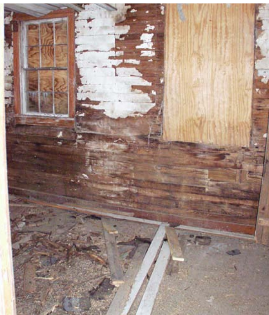
Figure 24 View south in Room 201. (NPS-SERO-CRS, 2001)
