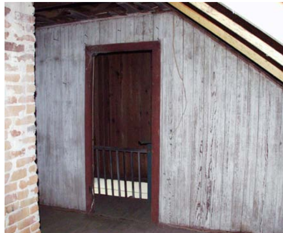
Figure 27 View south in Room 202. (NPS-SERO-CRS, 2002)
