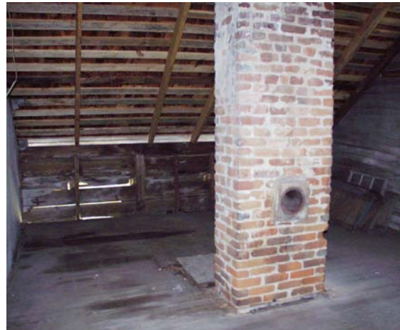
Figure 26 View west in Room 202. (NPS-SERO-CRS, 2002)
