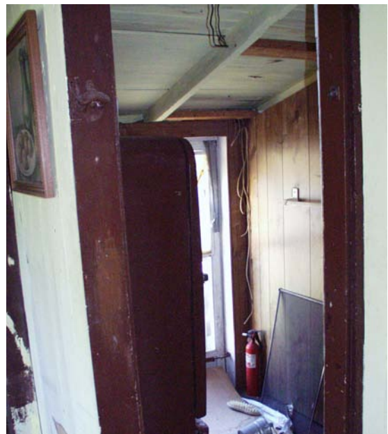
Figure 40 View to north of Room 105. (NPS-SERO-CR, 2003)
