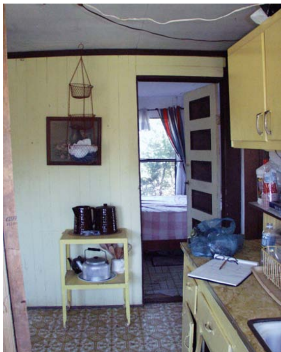
Figure 37 View northeast in Room 103. (NPS-SERO-CR, 2003)
