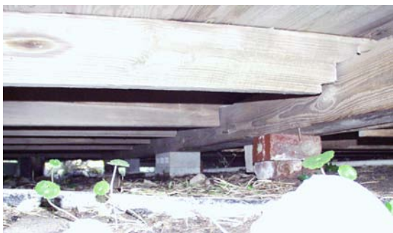
Figure 20 View west under Room 101. (NPS-SERO-CR, 2003)
