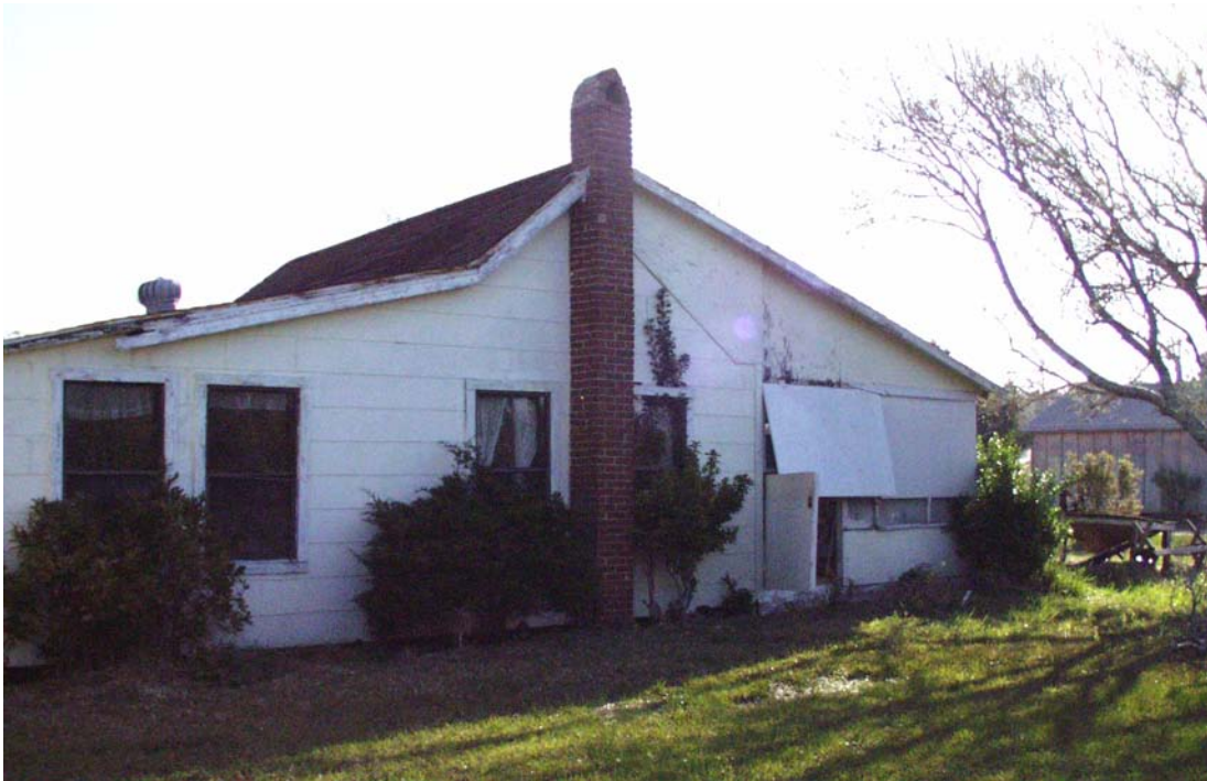
Figure 17 View east of house. (NPS-SERO-CR, 2003)
