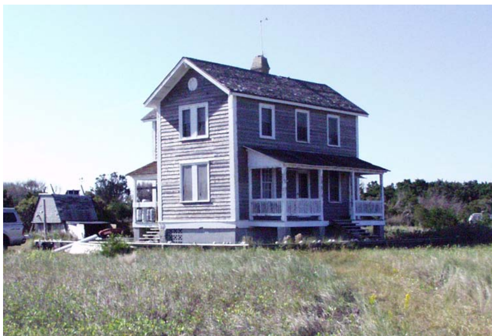
Figure 1 View to south of Barden house. (NPS-SERO-CR, 2002)
