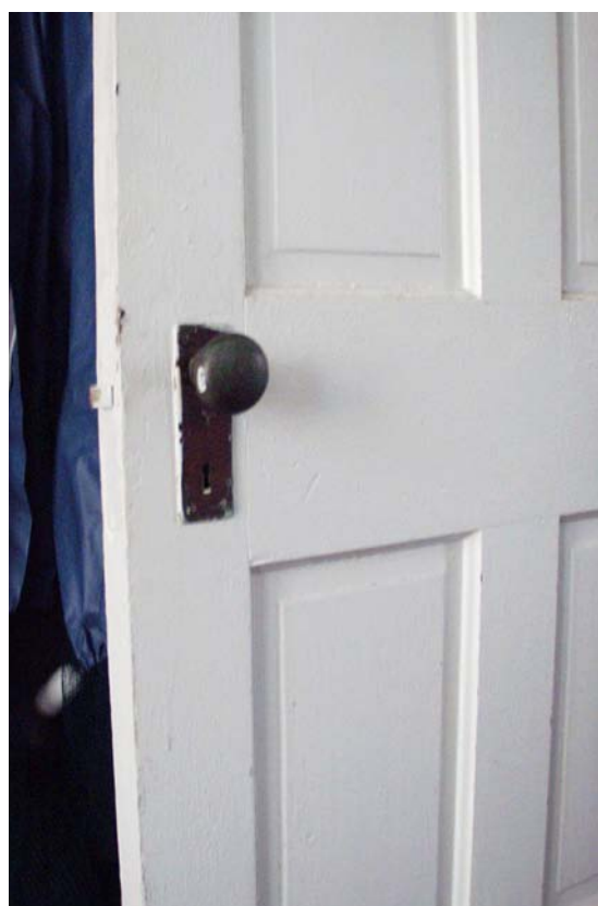
Figure 21 Detail of closet door in Room 101. (NPS-SERO-CR, 2002)
