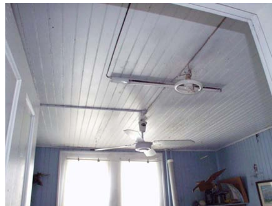
Figure 24 View of ceiling in Room 102. (NPS-SERO-CR, 2002)
