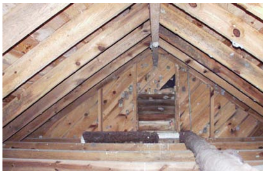
Figure 7 View southeast in attic. (NPS-SERO-CR, 2002)
