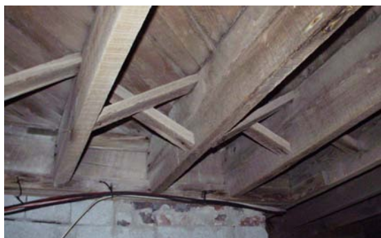
Figure 6 View of typical floor framing. (NPS-SERO-CR, 2002)
