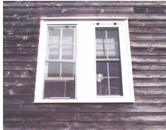
Figure 9 View of typical double windows. (NPS-SERO-CR, 2002)
