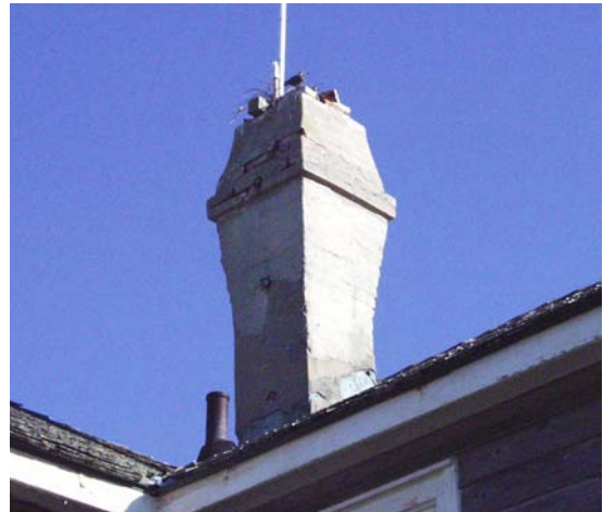
Figure 4 View of chimney. (NPS-SERO-CR, 2002)
