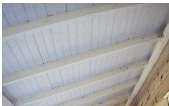
Figure 16 View east of front porch ceiling. (NPS-SERO-CR, 2002)
