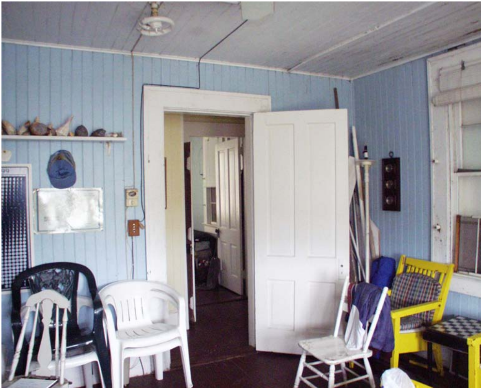
Figure 23 View to west in Room 102. (NPS-SERO-CR, 2002)
