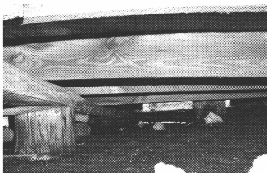
Figure 23 View of crawl space and piers. (NPS-SERO-CR, 2002)
