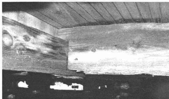
Figure 24 View of typical joist sill connection. (NPS-SERO-CR, 2002)
